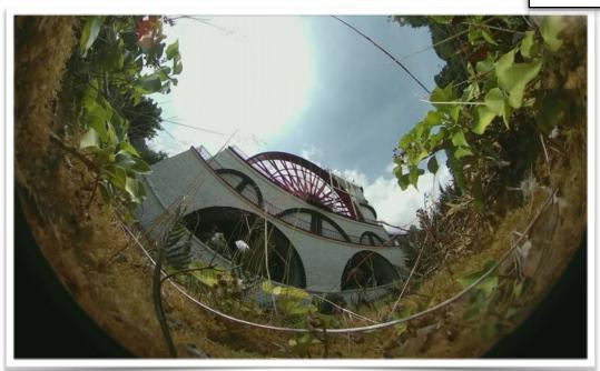
Designed by Robert Casement, the wheel has a 72-foot-6-inch (22.1 m) diameter, is 6 feet (1.8 m) wide and revolves at approximately three revolutions per minute.
